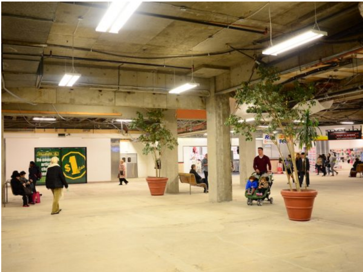
shopping centre basement concourse under renovation
