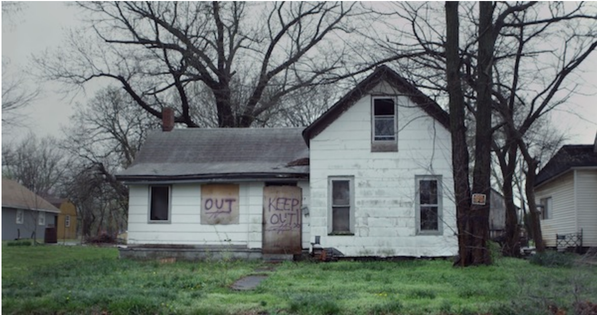
Boarded up home, Rich Hill, Missouri. Photo courtesy of "RICH HILL."
